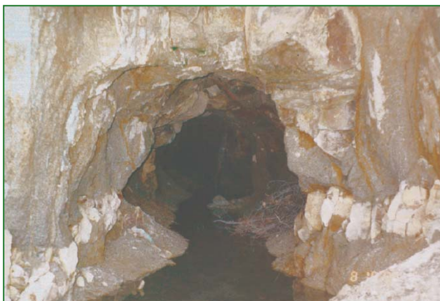
Figure 14—The lower (west) adit of the Charter Oak Mine discharges 0.4 to 10 gallons of water per minute. The extent of the workings and their relationship to other workings could not be determined.
