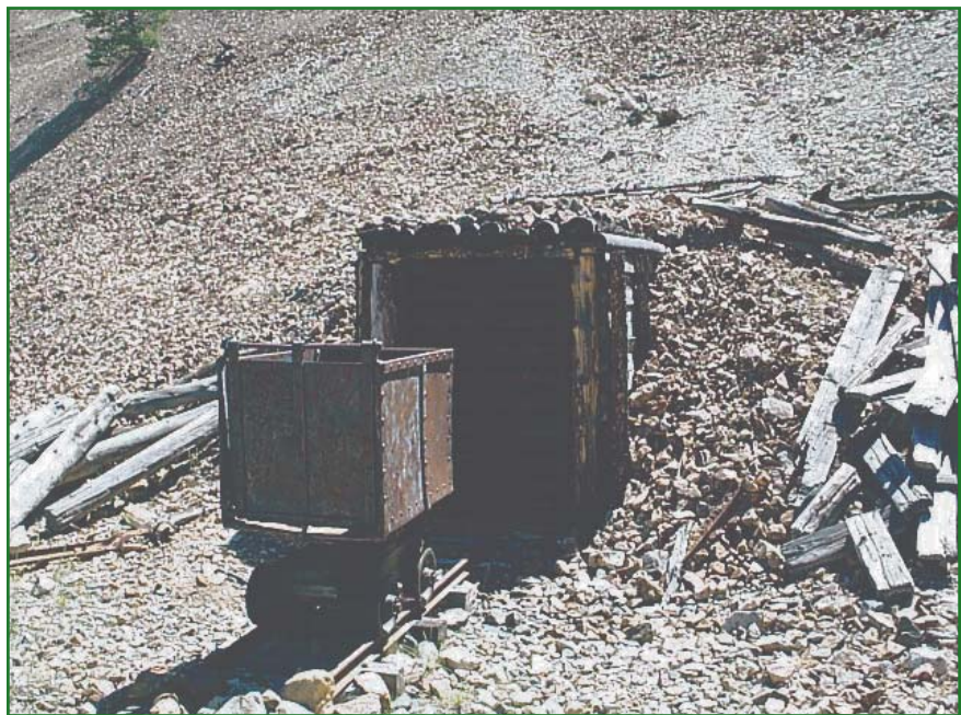
Figure 16—The main adit of the Charter Oak Mine is just uphill from the mill. A small discharge flows from the portal (entrance) and infiltrates the coarse material near the portal.
