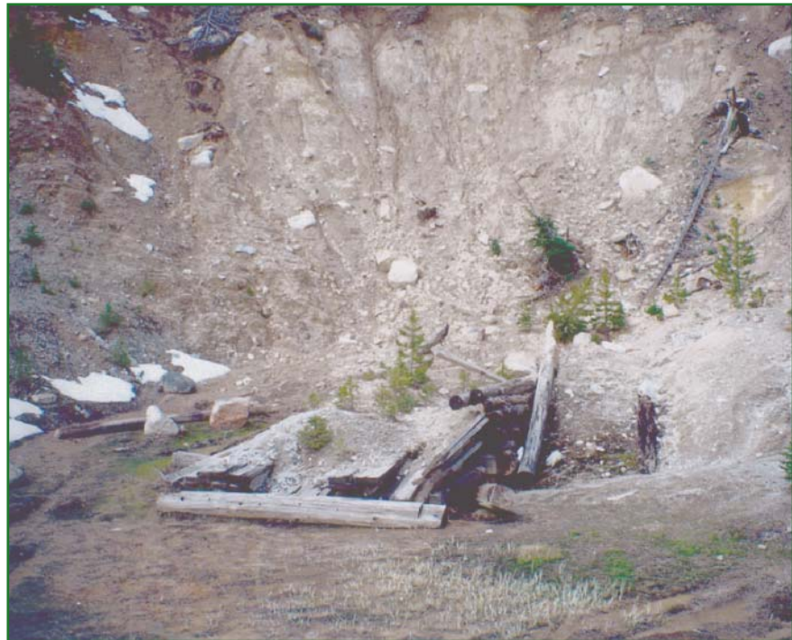
Figure 5—The upper Elkhorn shaft/adit (center of photo with lumber over it) discharges a small amount of water throughout the year.
