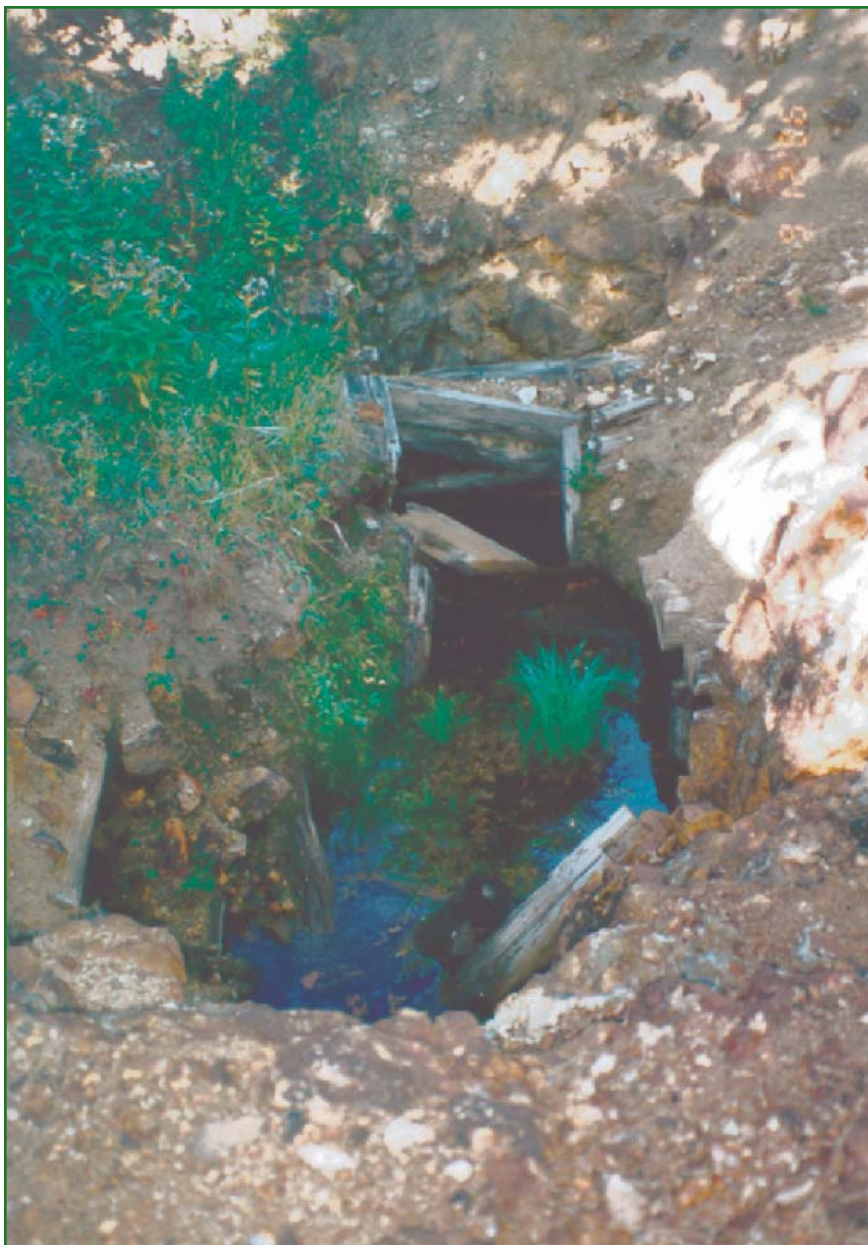
Figure 6—The workings at the Park Mine include a flooded shaft and several flooded cuts and prospects. The area is especially wet during snowmelt, but the workings are flooded throughout the year.
