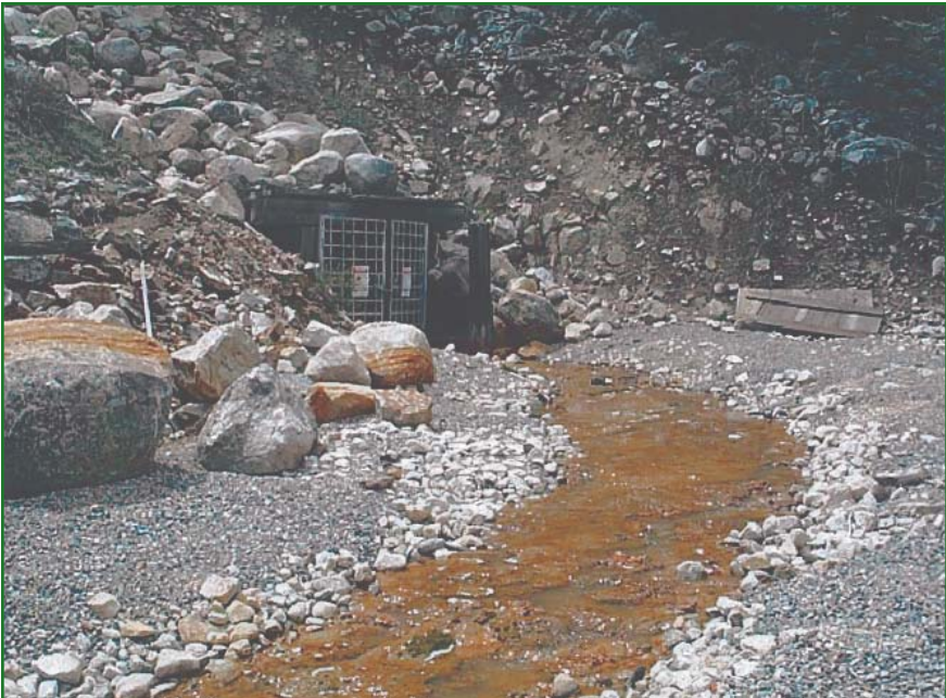
Figure 3—The discharge from the lower Elkhorn Mine adit ranges from 80 to 135 gallons per minute. The discharge stream eventually reaches Elkhorn Creek, a tributary to the Wise River.
